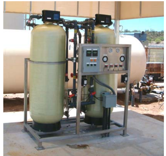
Use of E33 media in typical Modular and APU system installations.
