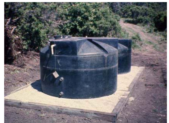
Large residential project treating creek water with two 5000 gallon storage/contact tanks.
