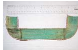
Section of corroded copper pipe. This customer had pinhole leaks in the copper piping caused by acidic water.
