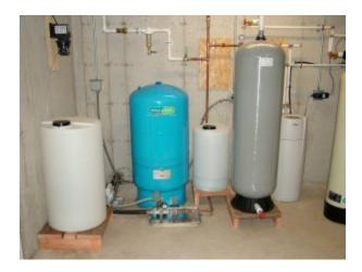
To make up a 10% solution mix 4 lb of soda ash powder for every 5 gallons of water, which is approximately a 10% solution by weight. It is best to use warm purified distilled or reverse osmosis water to make up your solution, although if your untreated well water is very low in total dissolved solids and other minerals, you can generally use the untreated water to make up the solution.
