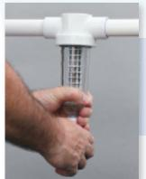
Accessing the filter is a wet and dirty mess. Depressurizing the system introduces air into the system.
